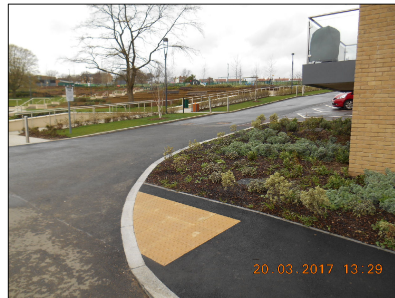
DETAIL 1 - TACTILES WITH ASPHALT SURROUND
