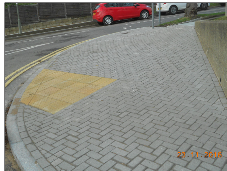
DETAIL 2 - TACTILES WITH BLOCKWORK SURROUND
